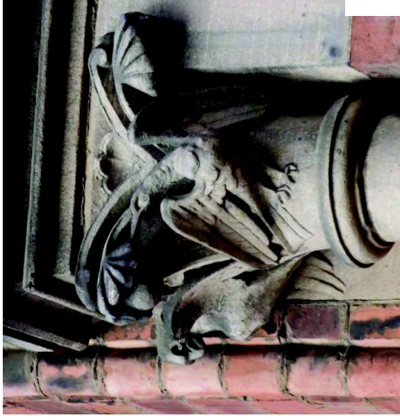
Wenlock Terrace – typical column head
